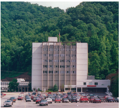
Elliot Building Completed
